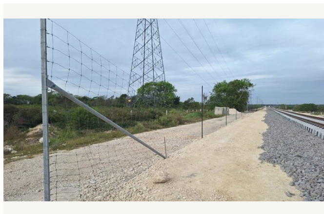
Perimeter enclosure alongside the railway.
