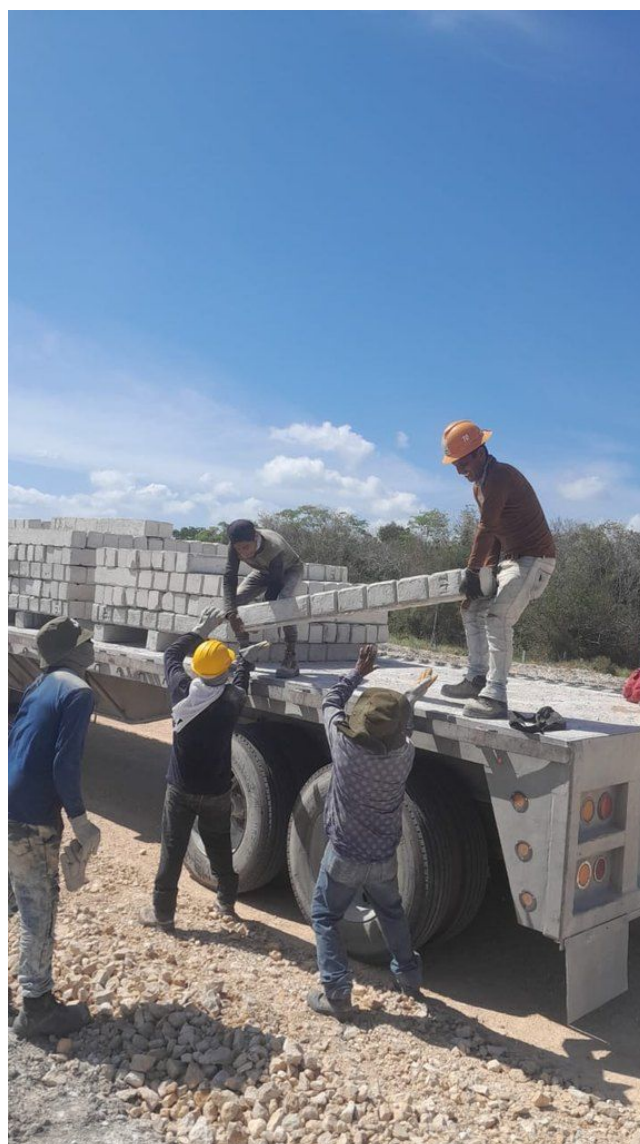
Unloading posts at the work front.
